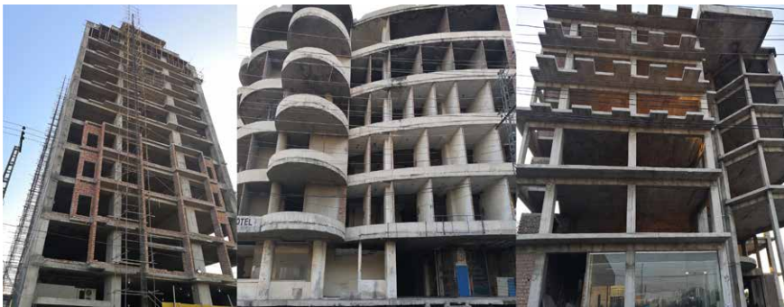
Figure 91 Under construction projects
